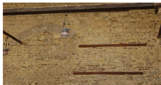
Figure 1 Construction system of the double faced masonry walls in Islamic monuments in Cairo.
