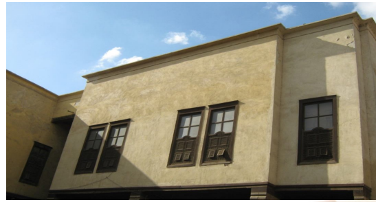
Figure 7 Present state of Wkallah Radwan Al-Fakari, before restoration processes.
